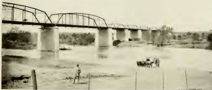
THE SAN JOSE ROAD BRIDGE.
